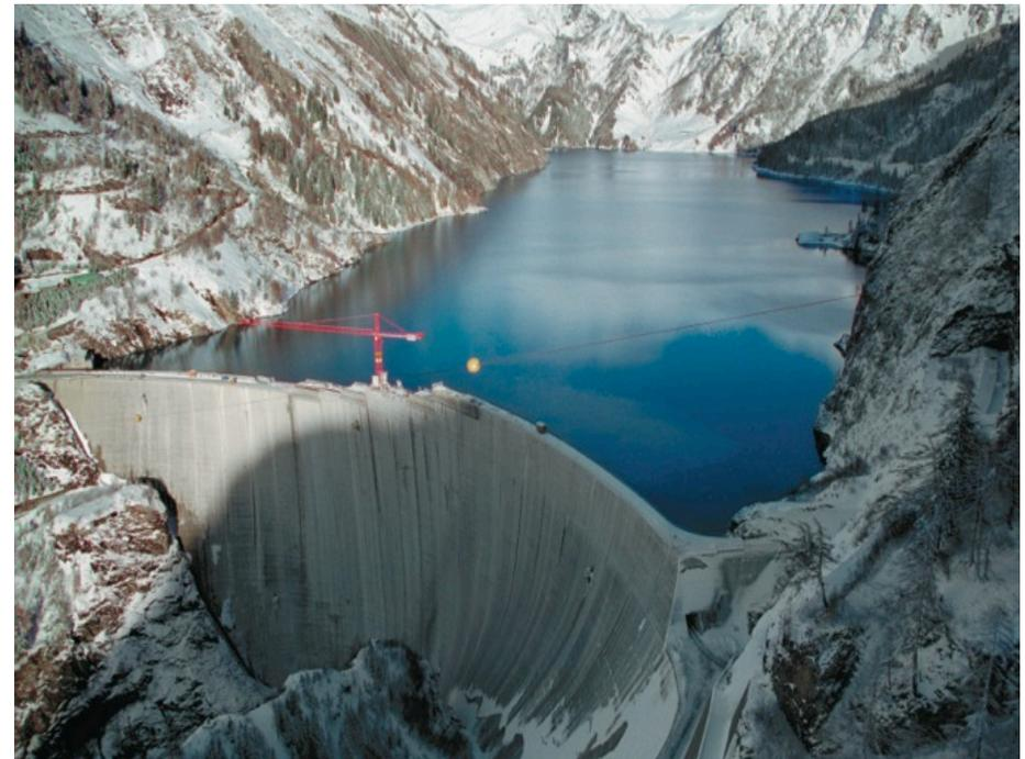
Heightening of Luzzone dam from 208 m to 225 m (TI) 1995 - 1999
