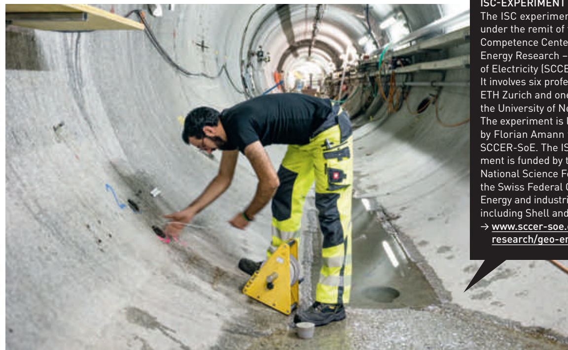
Team member Reza Jalali carefully feeds a fibre-optic cable into a borehole.
