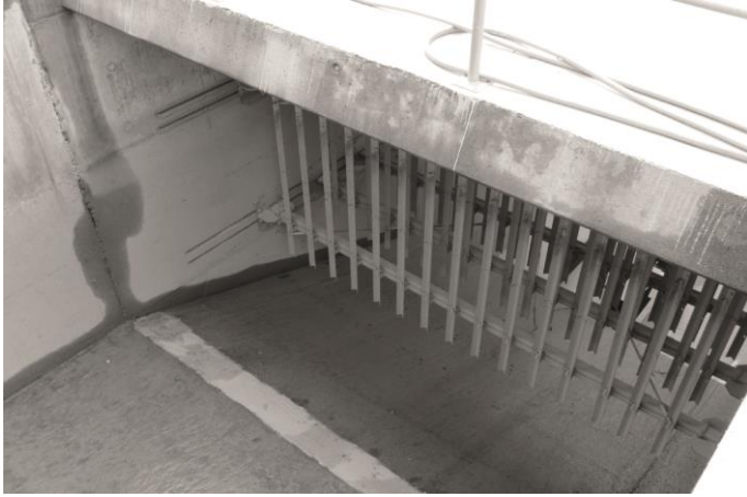
Figure 16. Three rows of tranquilizing racks with V-shaped bars (tips pointing downstream) upstream of the basin at Wysswasser. Source: VAW.
