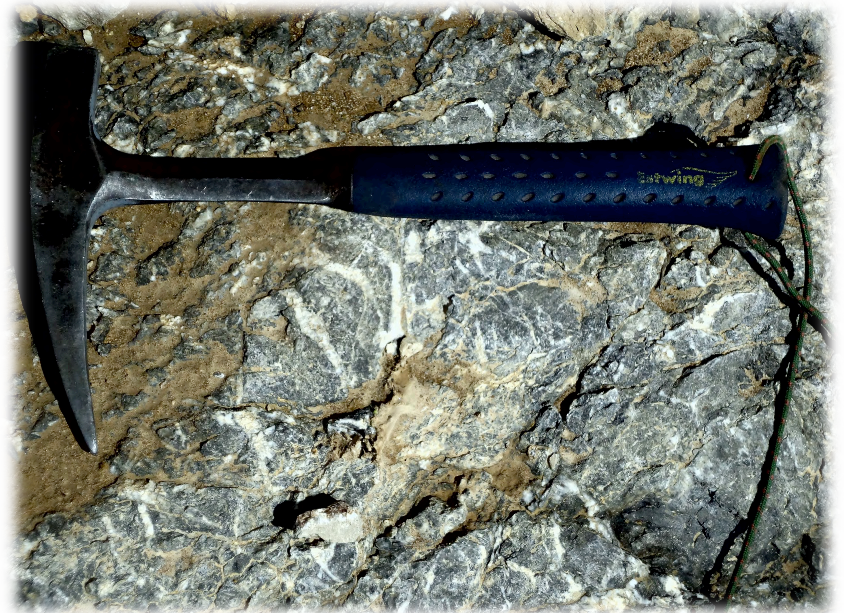
Figure 2: Detailed view of the damaged fault core with brecciated and heavily veined limestones.
