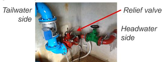
Instrumentation and data acquisition performed by hydraulic energy team of HES SO Valais
