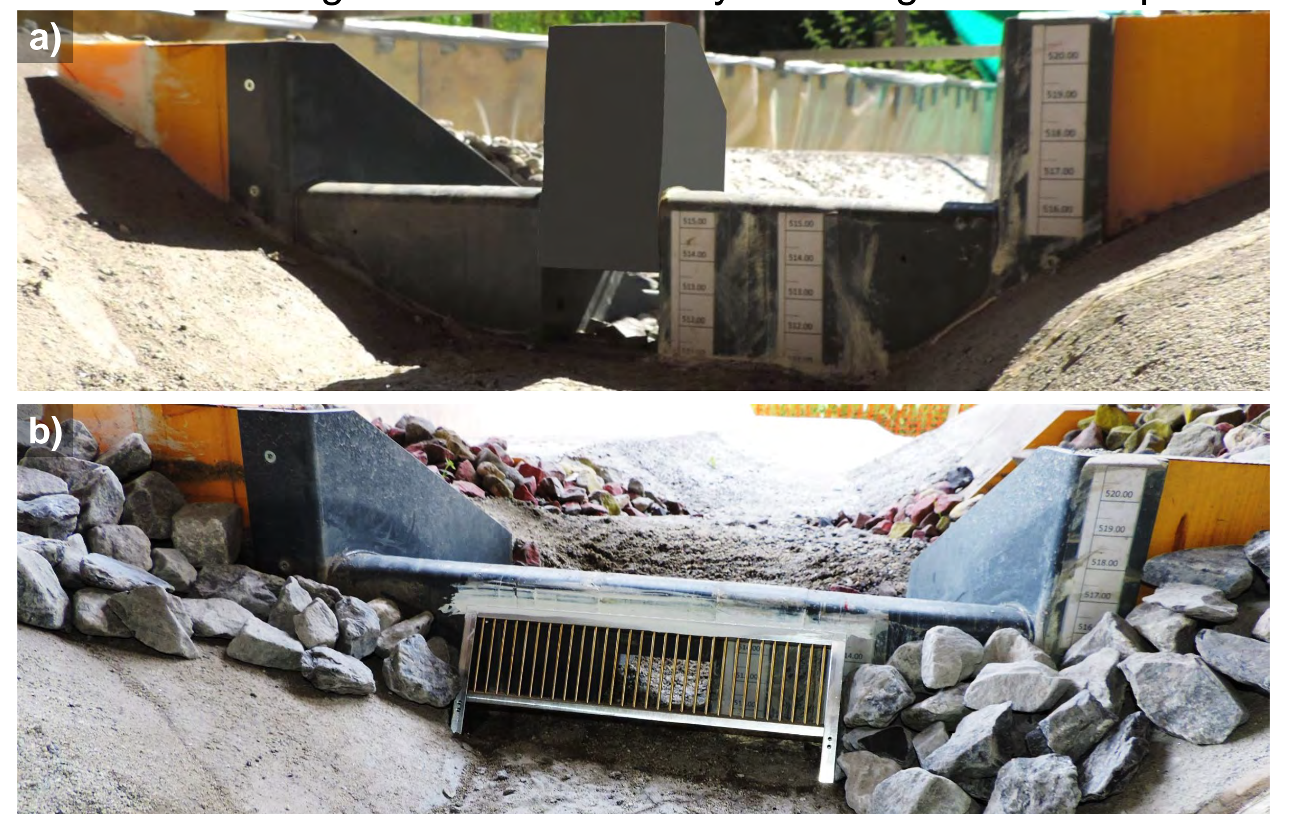
Figure 5: Illustration of a) the initial design of the filter check dam and b) the optimized design with screen for passive obstruction
