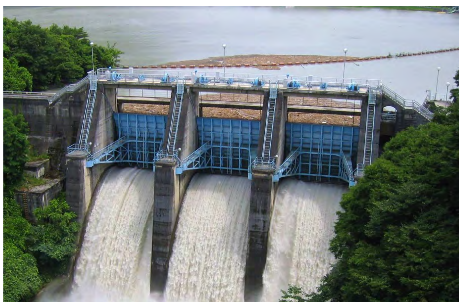
Figure 1: Picture from downstream of Takato Dam, Japan. Upstream of the gates it can be seen the accumulation of LWD (www.commonswikimedia.org)
