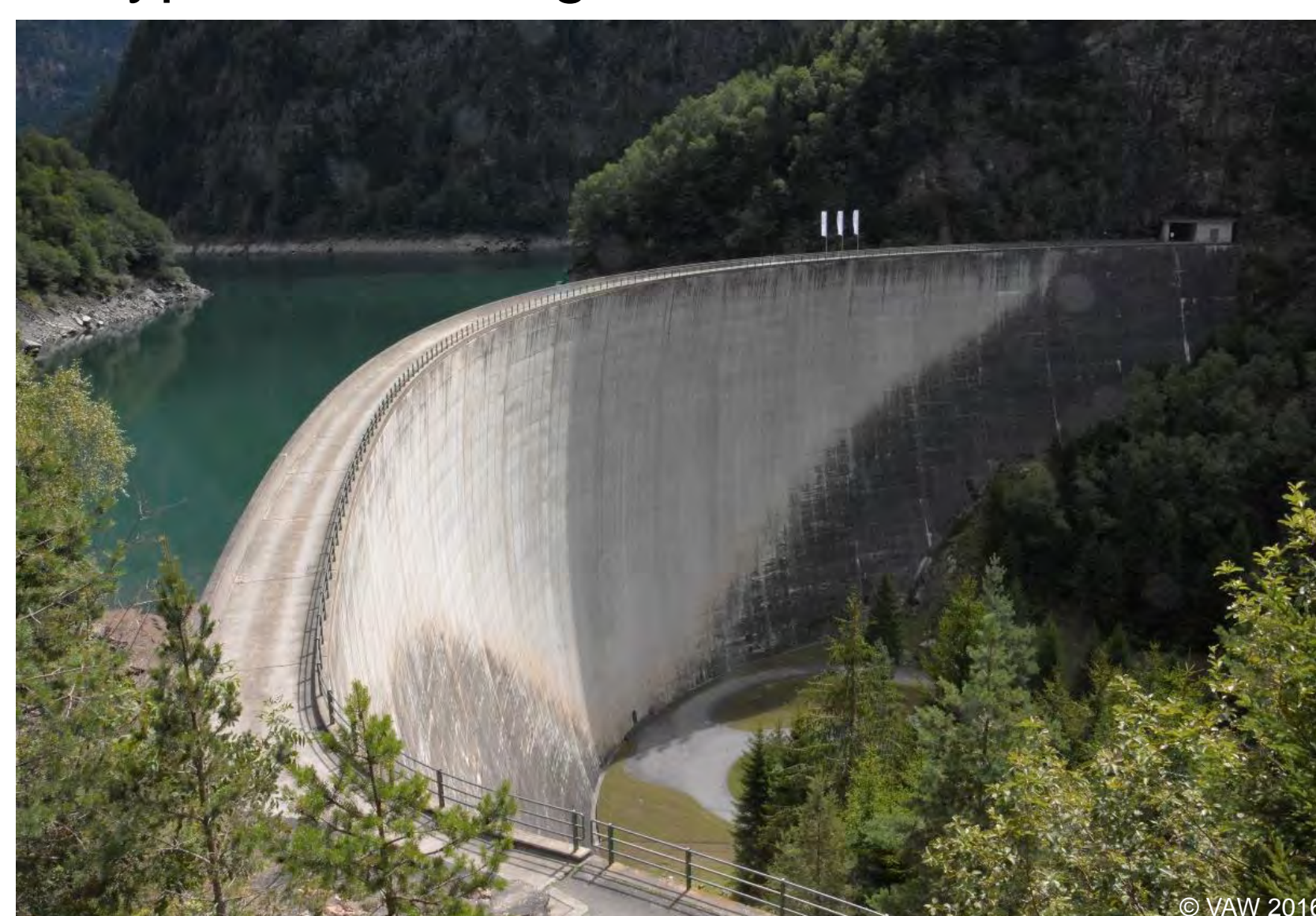
Fig. 4: Malvaglia arch dam
