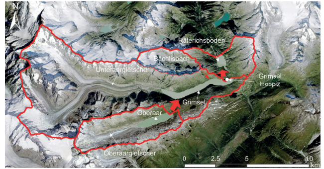
Figure 1 Aerial view of the system formed by the reservoirs of Oberaar, Grimsel, and Räterichsboden
