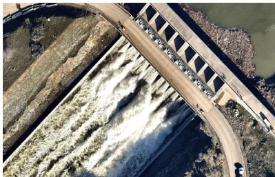
Figure 1: Picture of Oroville Dam, USA. (www.sacbee.com)
