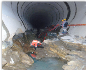
Fig 1. Hydro-abrasion at Palagnedra SBT (Photo: VAW, ETH)
