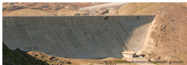
Fig. 2: Arch gravity dam Gries
