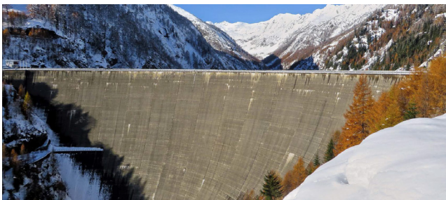
Fig. 1: Downstream view of Sambuco arch gravity dam.
