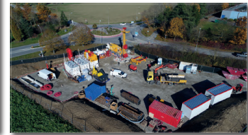
Aerial view of the GEO-01 Drilling site
