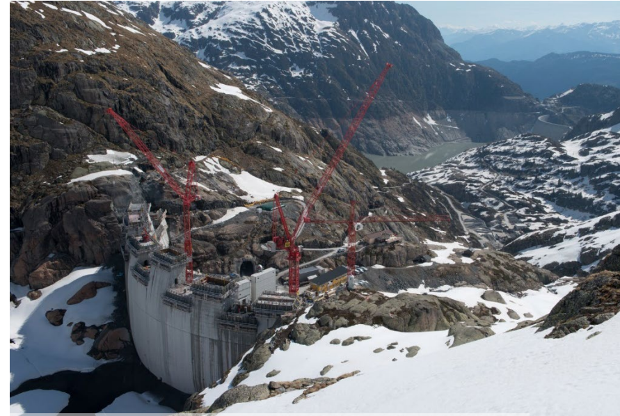
Heightening of Vieux Emosson dam (2012-2015) by +21.5 m (39%) → +93% in volume
